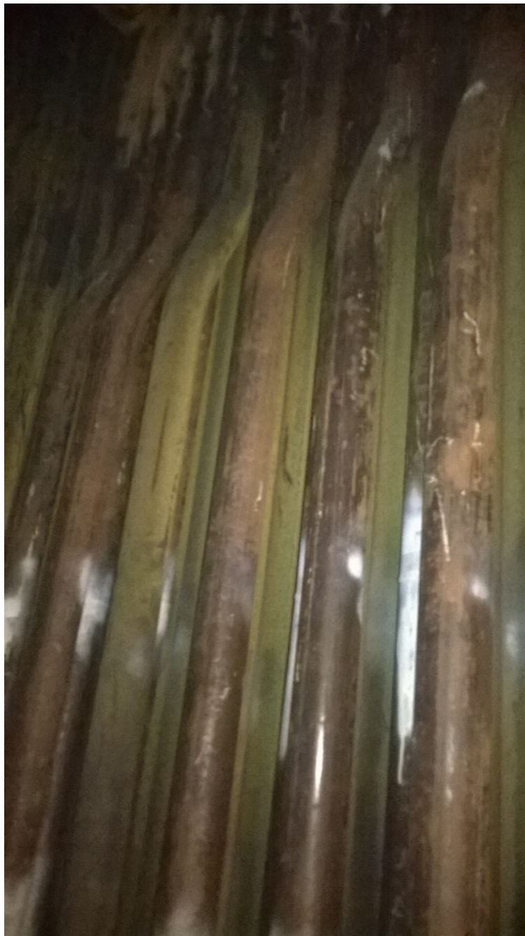
Figure 4: Installation of Screen tubes
