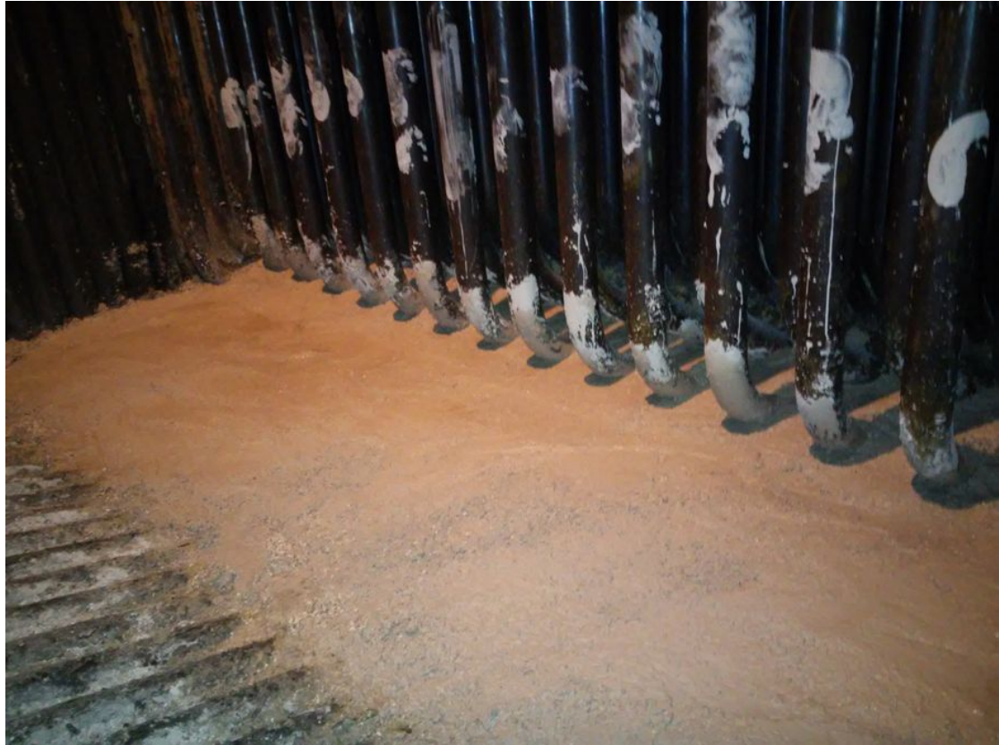
Figure 3: Installation of refractory
