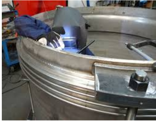
Figure 16: Fabrication of Expansion Bellow
